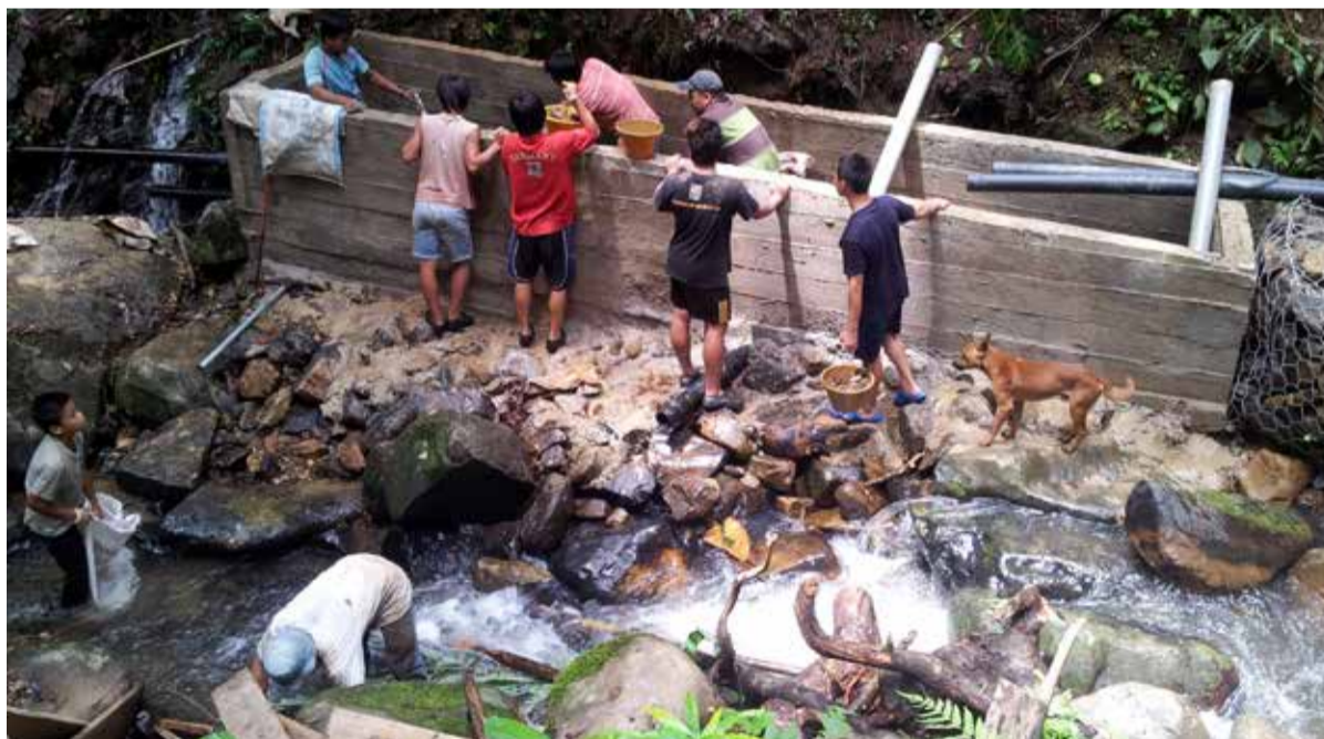
Building the reservoir tank.
